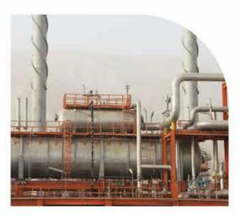
The enhancement of thermal efficiency is the other benefit of using it. The deaerators can bring down the oxygen content of the boiler feedwater to 7ppb. ASME, ASTM, and HEI are standards according to which these products are being designed and constructed in the company.
